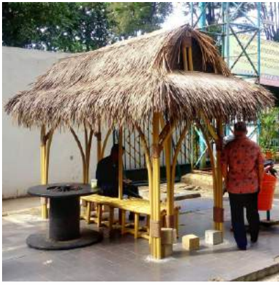
Saung/Gazebo, built from Virobamboo and Virothatch at parking lot a university in Jakarta.
