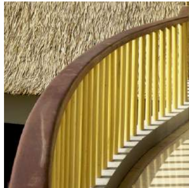
Virobamboo installed as railing balcony.
