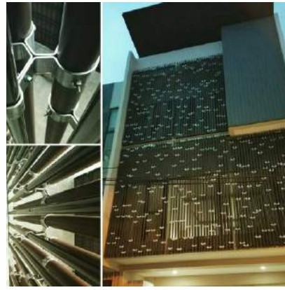
9- Parametric Y-Clamp Modular Joint System uses Virobamboo for building facade, designed by Formologix.
